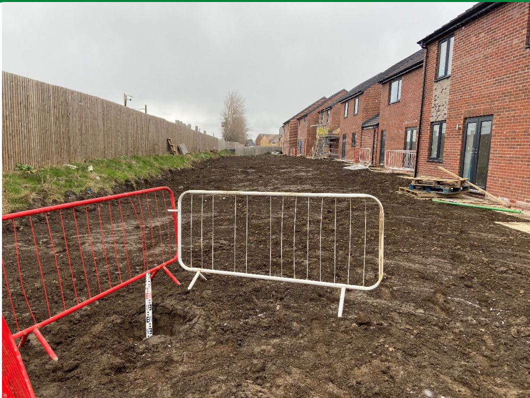
PLATE 2 – SHOWING GENERAL PLACEMENT IN PLOT 67
